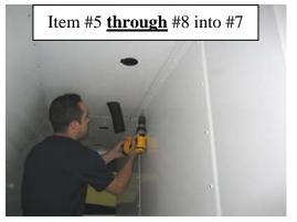
Pre-drill through **Ceiling** sections, (using **Divider** as a template), with 3/16" drill bit and attach using ½" x 1 ½" hex head lag bolts
